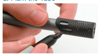
Position the Rynglok Marking Gage (P/N: RTSG0-01-XX) on the end of the cut tube. Use a suitable marking pen to make the position and inspection marks.
